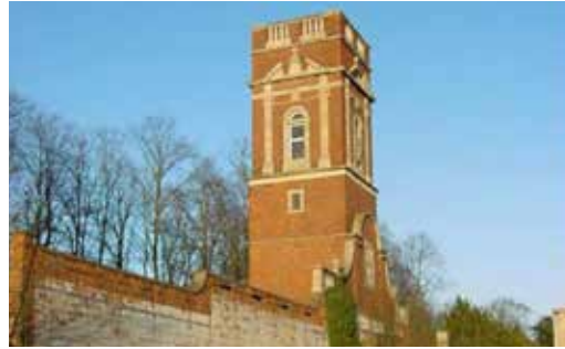
View 2. Water Tower
