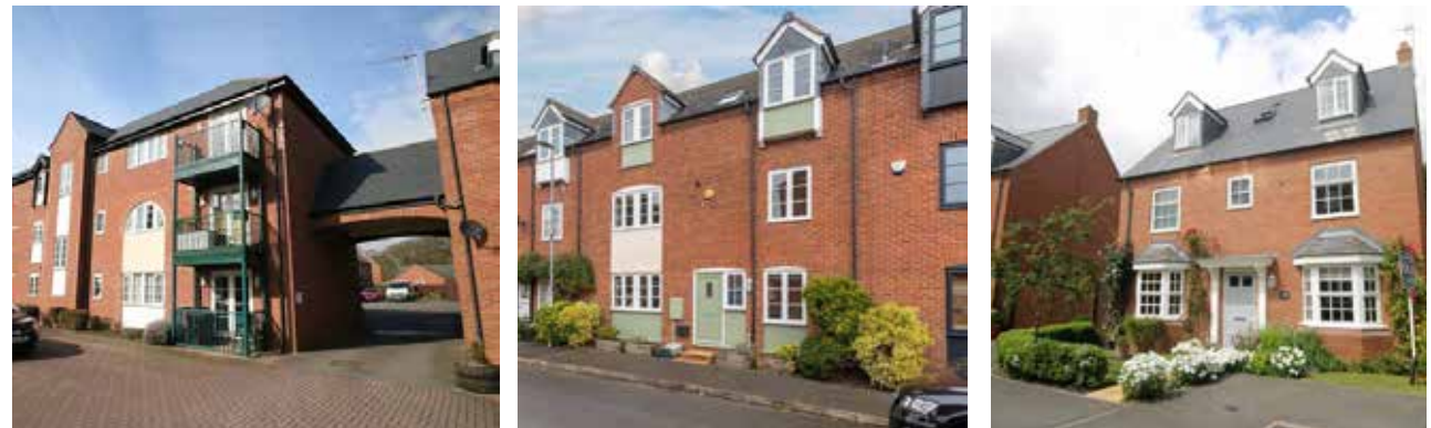
Figure 36: View of typical streets and building typologies in the Post-2000 Development Character area
